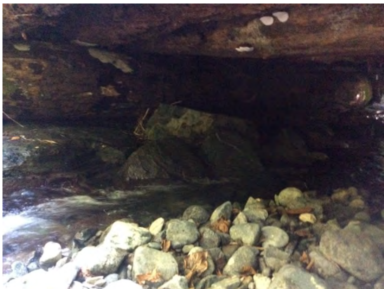
Left Bank Abutment when facing downstream
