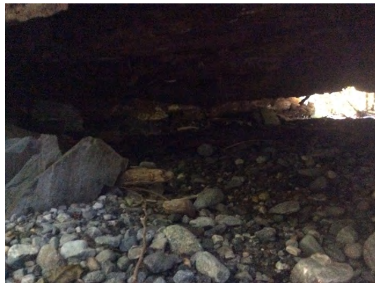
Left Bank Abutment when facing downstream
